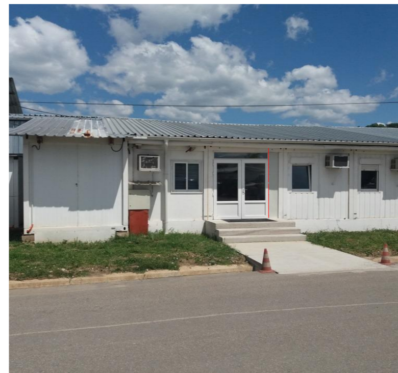
Existing entry in Block#6 as example
