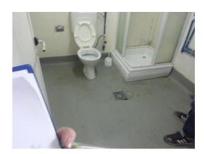
The new floor Gully Drainage of stainless steel dim. 200x200mm with 50mm OD outlet is to be installed in all small ablution units. The old gullies are to be dismantling and the opening is to be adjusted for the new gully.
